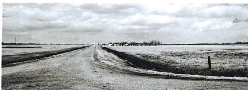
Many rural residents think the road ditch is to improve drainage on their property. However, the ditch is there to improve drainage on the ROAD.
